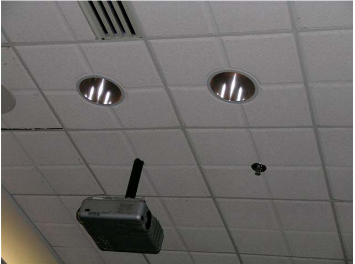
Standard tegular ceiling tile custom cut around ceiling penetrations.
