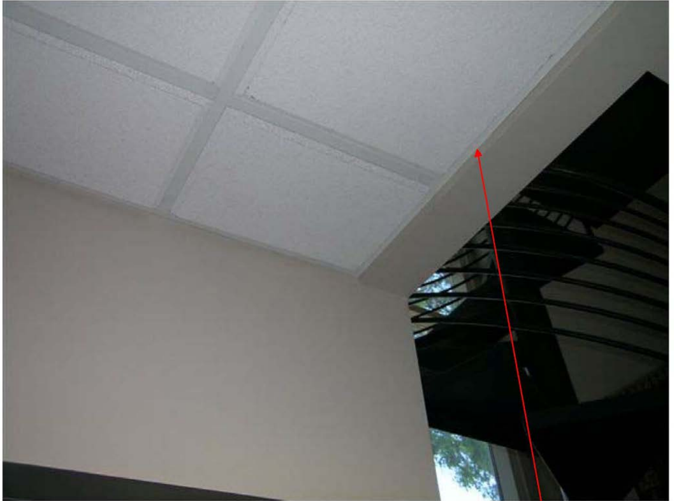
Standard Lay-In Ceiling Grid / drywall bulkheads
