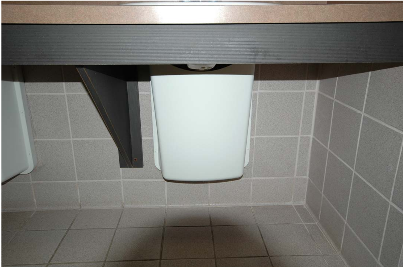
Preferred pipe enclosure installation in knee space below vanity.
