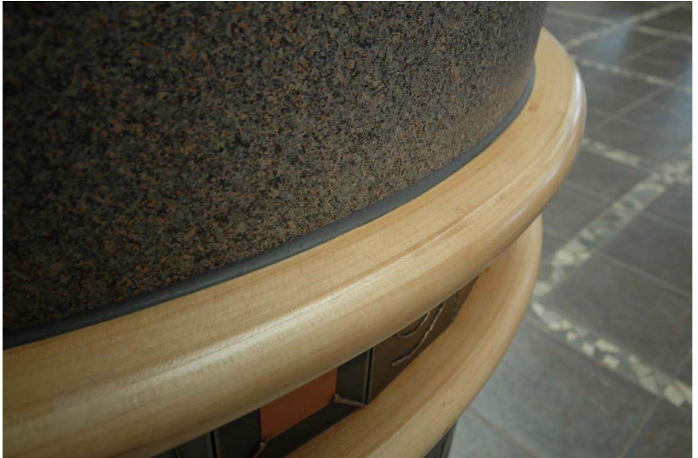
Caulk joint installation Small, consistently sized, smooth joint
