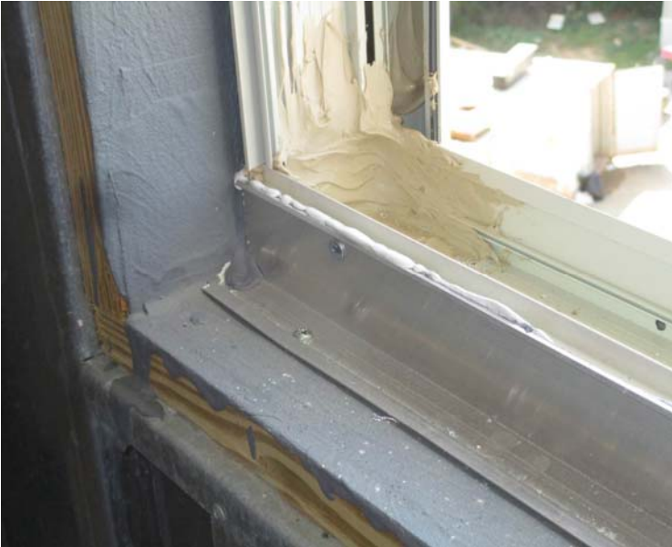
Figure 3: Interior side of an interior trim angle with receptor installed. Fasteners must be cap sealed. It is the contractor's responsibility to ensure compatibility of sealants to LAMF and fenestration products.
